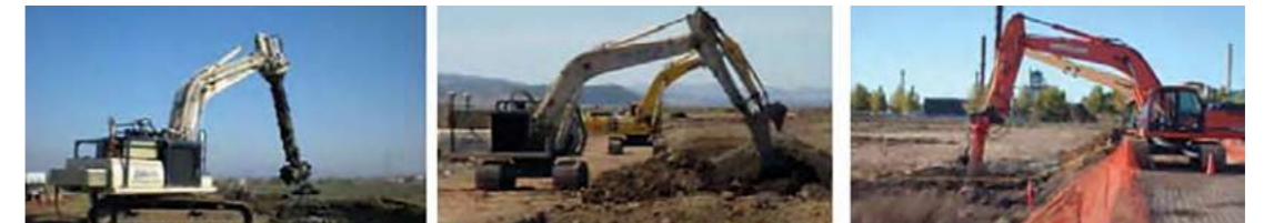
In situ stabilisation of sediment and soils impacted with Hg and PAHs in a former effluent treatment pond using binder agents. Source: ARCADIS
