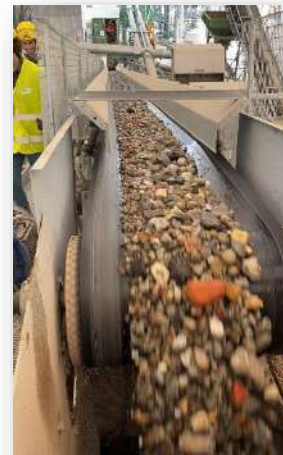
Figure 1.3 - Soil washing stage conveyor belt
