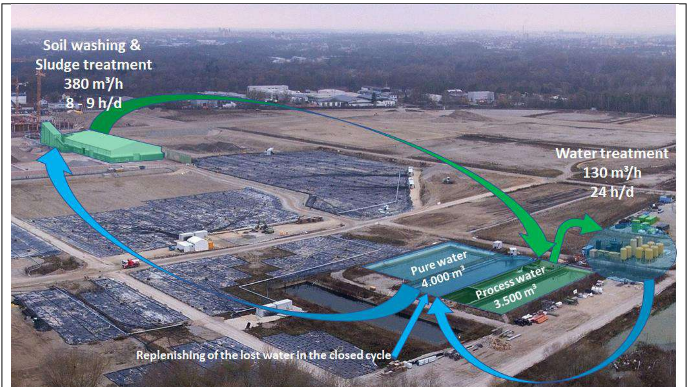
Figure 6: Water management using large basins to reduce the capacity of the water treatment plan, Copyright: ARGE AUDI IN-Campus GbR. The water treatment units purifies approximately 140 m 3 /h of clear water, removing the dissolved contaminants with sand filters and activated carbon. Depending on the contaminations at hand, different types of activated carbon are employed to optimize the adsorption capacity. A share of the washing fluid is lost by adhesion to the output soil, and needs to be replenished with fresh water (external supply).
