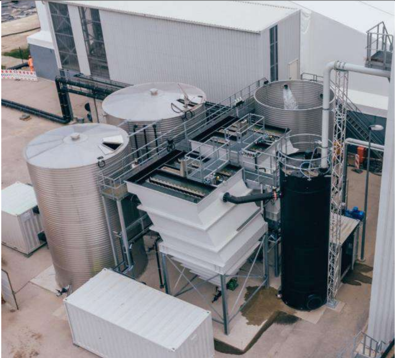
Figure 4: Areal view of the sludge treatment plant, Copyright: ARGE AUDI IN-Campus GbR.
