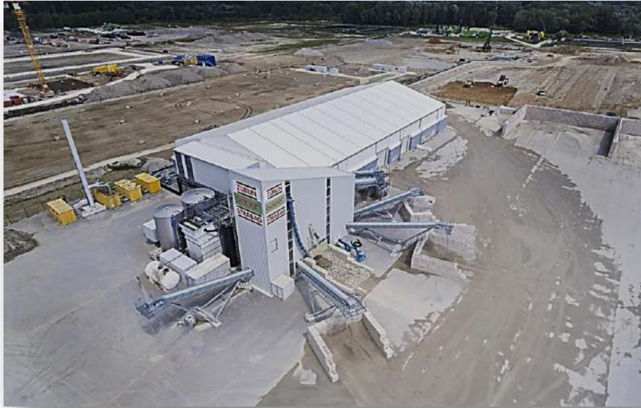
Figure 2.3- Areal view of the soil washing plant (front), sludge treatment facility (left hand side) and the reception hall (in the back). Copyright: ARGE AUDI IN-Campus GbR (ask for permission to Dr. Benjamin Faigle – Züblin Umwelttechnik GmbH)
