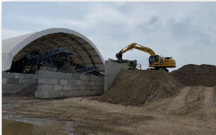
Figure 1.2- Contaminated soil loading area
