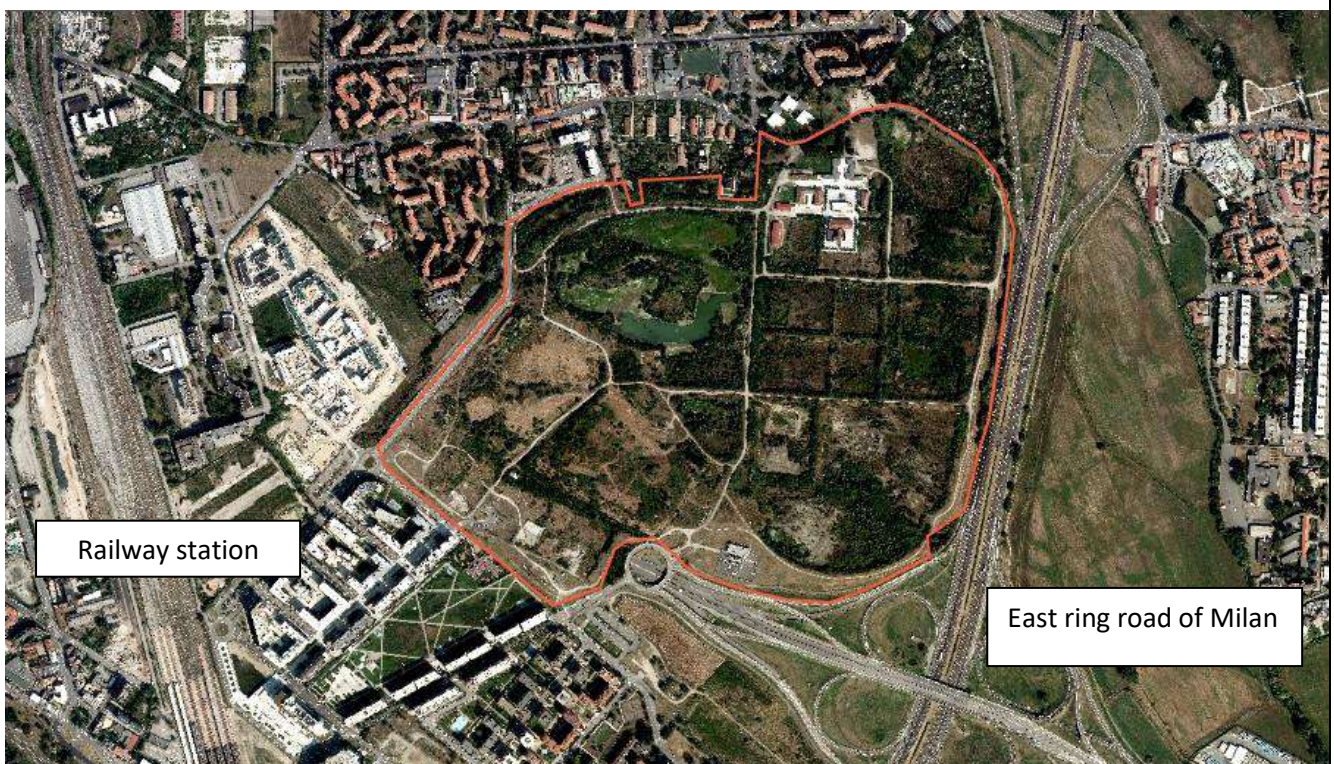
Figure 11 - Location of the contaminated site (in red), with respect to the railway station and the eastern ring road of Milan
