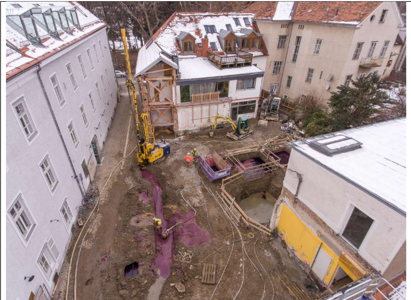
A picture of the site. Works are conducted below former washing machines. Backflow deeply covered purple by \text{KMnO}_4
