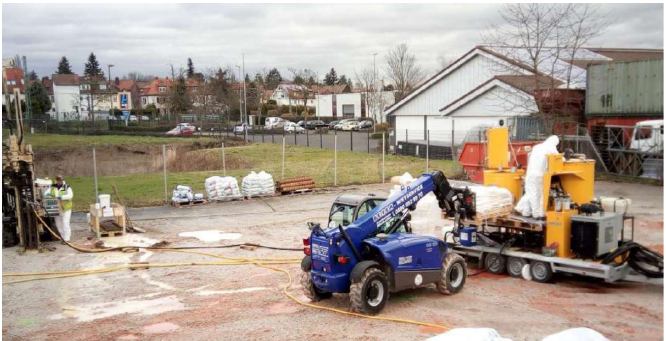
High pressure injection/fracturing/ and mixing equipment used for fracture-emplacment of persulfate-peroxide oxidant slurry into subsoils through direct push drill holes
