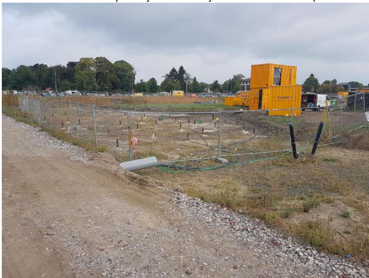
Overview injection filters in source zone
