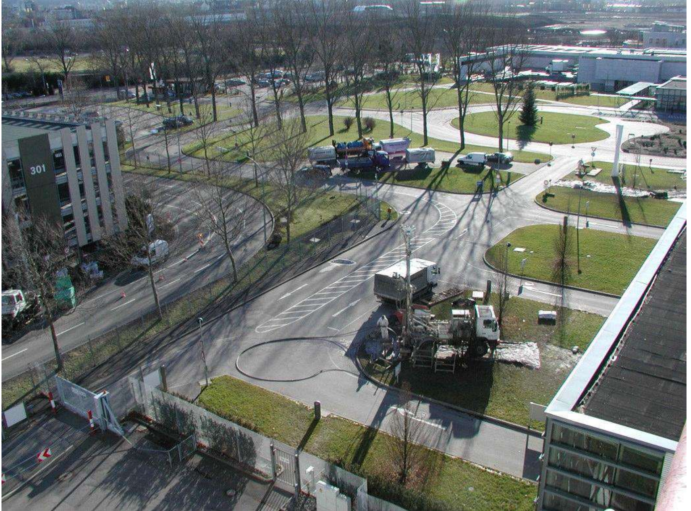
Drilling work for the remediation wells in front of building 25/1
