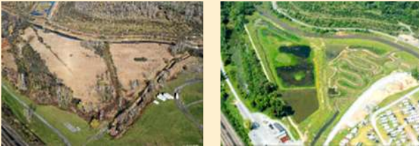
Geddes Brook Wetlands Before and After Remediation
