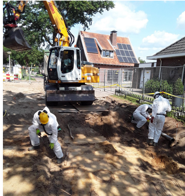
Removing asbestos contaminated soil | NTP
